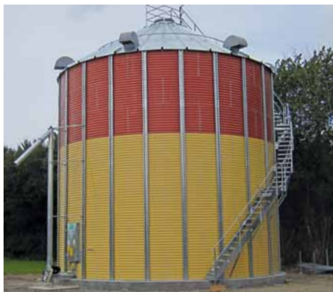
Silo installation with side sheets in two different colours and a galvanized roof.
